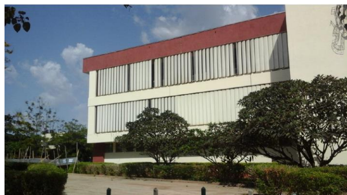
Figure 5: Horizontal shading devices used on the north face of the building.
